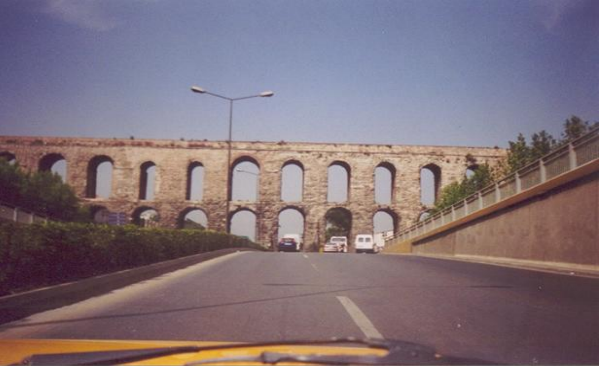
Section of the aqueducts built by Valens, as seen from driving into modern day Istanbul.
